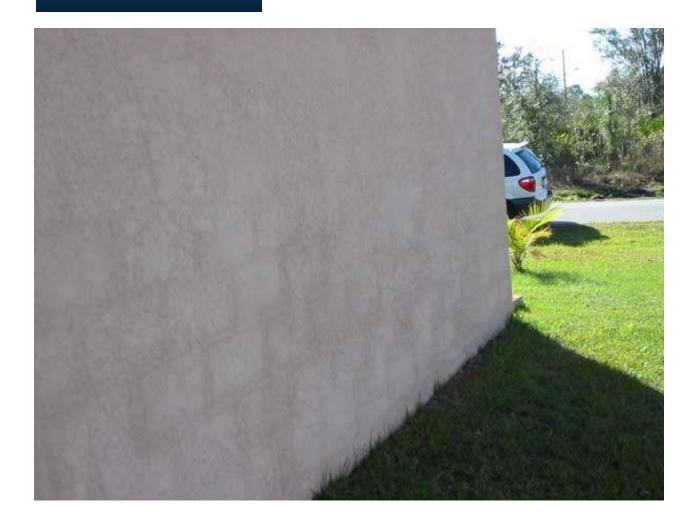
Factors affecting the ghosting phenomena include curing of the masonry wall, curing of the stucco, densification, and thickness of the plaster.
