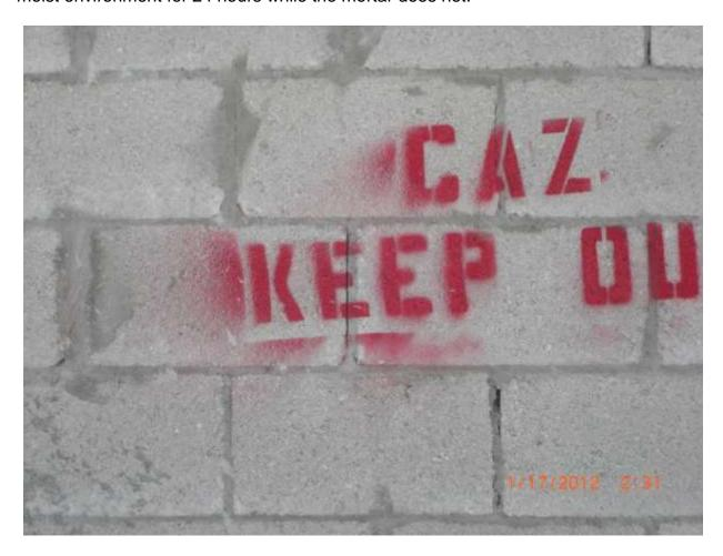
The crack above is due to mortar shrinkage. Sometimes these cracks will continue in a "stair step pattern following the mortar joint. Shrinkage cracks are very narrow (usually less than 1/32-inch) but will reflect through the stucco.
